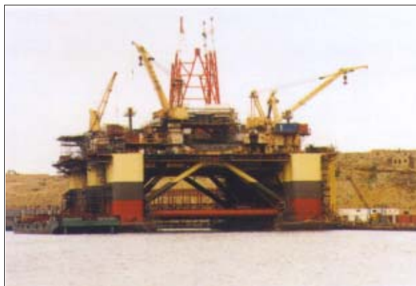
Upgrading existing equipment to Western technology standards.
