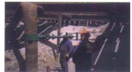
Hot Tapping 13 3/8" Casing.
