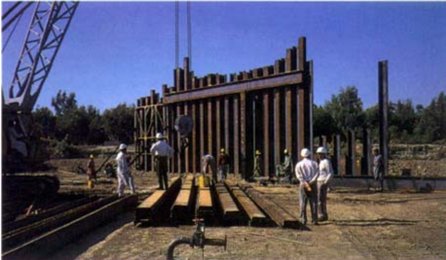
Cofferdam "Sheet Piling" Construction/Dewatering Well in foreground.
