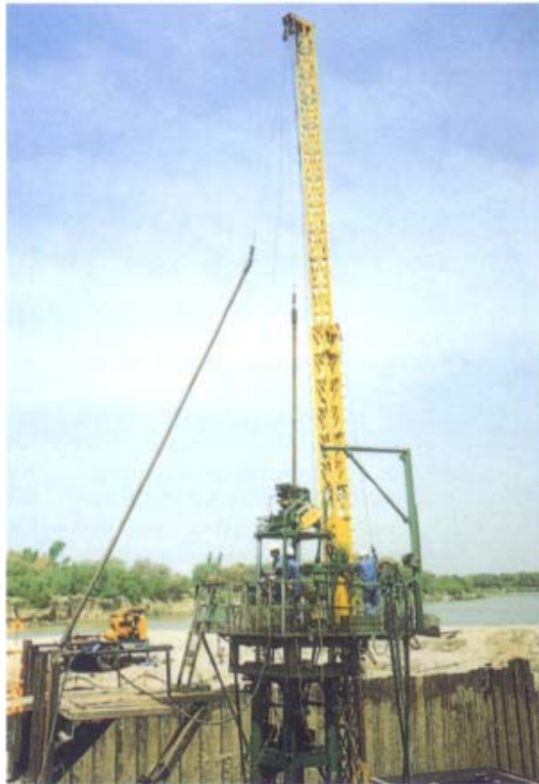
Hydraulic Workover/Snubbing Unit.
