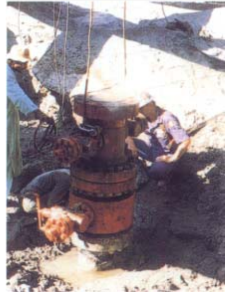
Removal of Casing Head.
