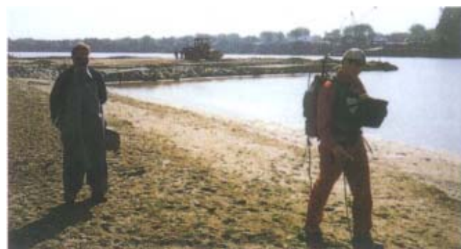
Ground Penetrating Radar along the initial berm construction.
